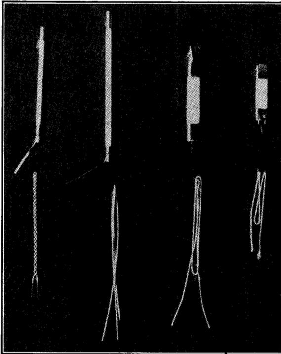
FIG. 2-6. Indirectly and directly heated cathodes used in high-vacuum receiving tubes.
